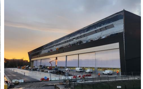
Mérignac – Multifunctional production facility
