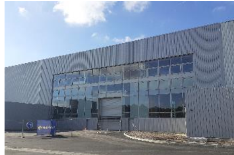
Martignas – Joining of Buildings 1 and 2
